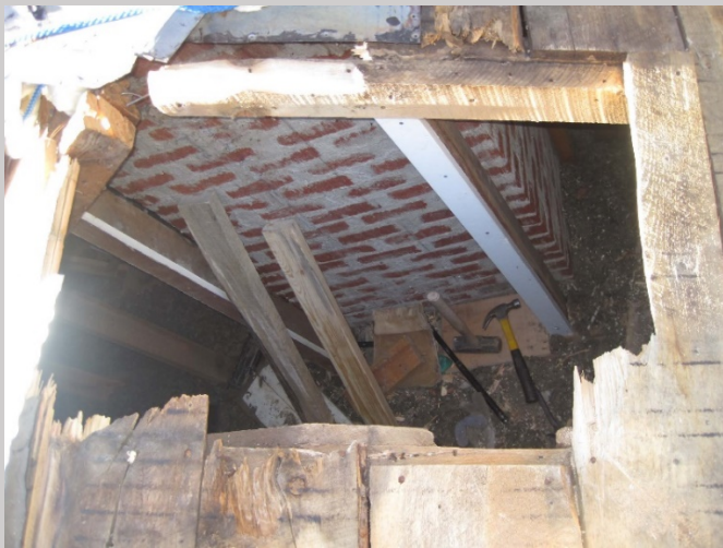
Photo E. The porch on the historic log house was reconstructed on the west side to remove its weight from the log wall, now resting on its own foundation. The south side was repaired. The lumber is rough sawn to be like the original. Logs were skidded to sawmill, cut into lumber and hauled to the site.
