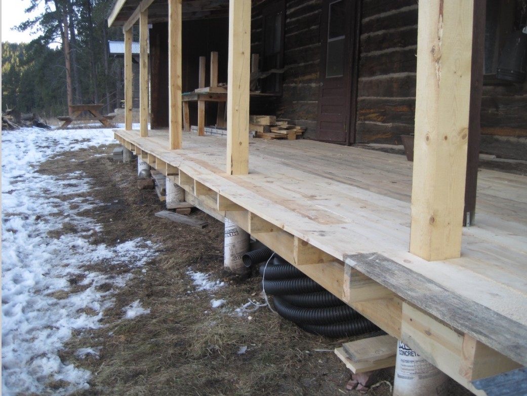
Photo E. The porch on the historic log house was reconstructed on the west side to remove its weight from the log wall, now resting on its own foundation. The south side was repaired. The lumber is rough sawn to be like the original. Logs were skidded to sawmill, cut into lumber and hauled to the site.
